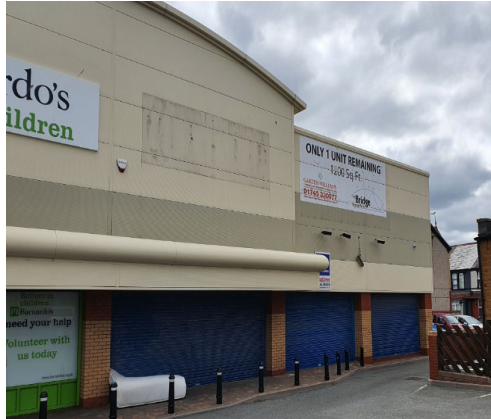
Units 2A and 2B
